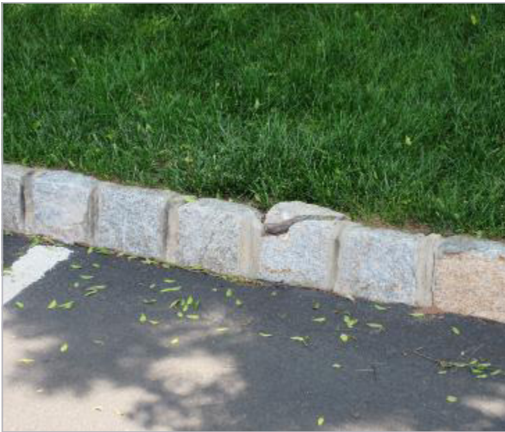
Photo Three— Chipped block in curbing along visitor parking area
