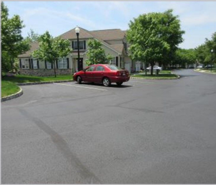
Photo One— Lateral cracks in pavement by visitor parking
