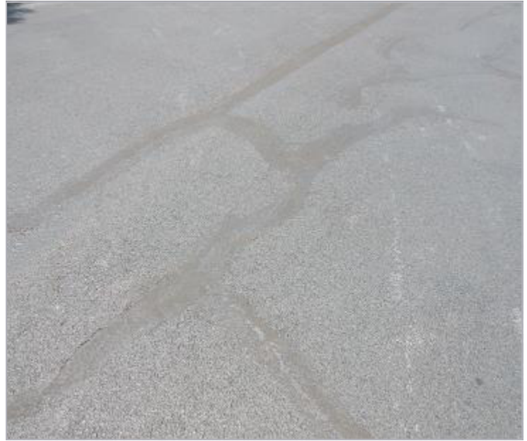
Photo Two—Spider cracks in pavement along W Hampton Way
