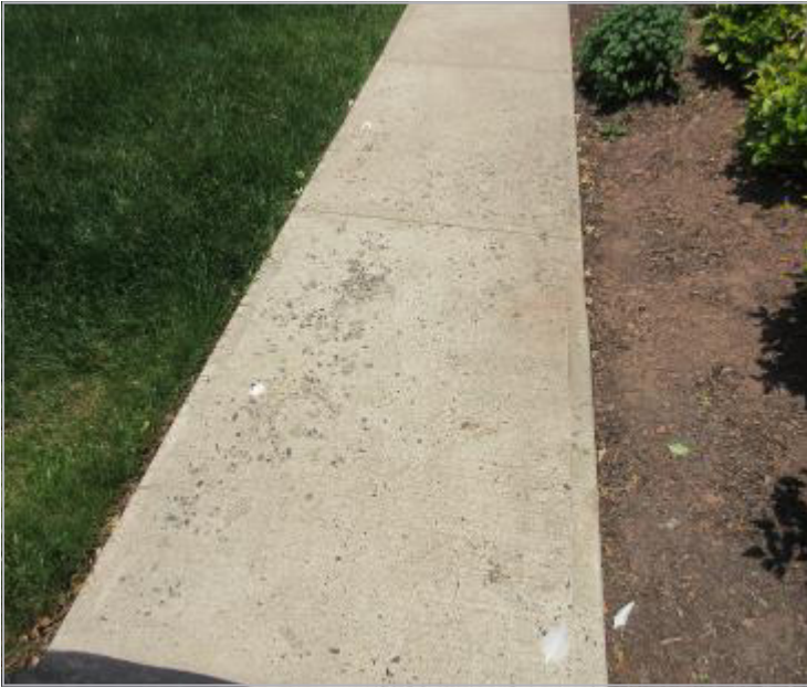
Photo Five— Spalling on walkway to Unit #37
