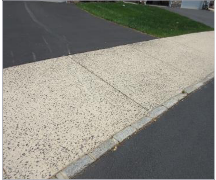
Photo Six—Spalling on driveway apron (typical condition)
