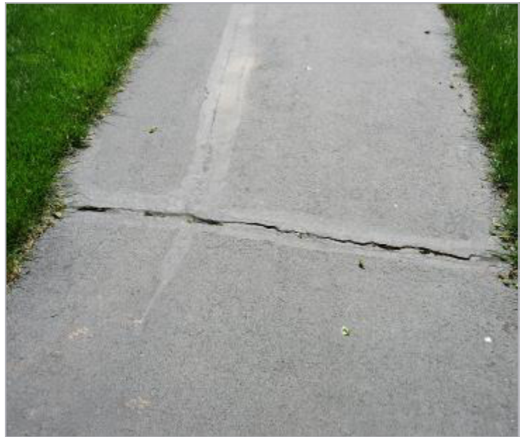
Photo Eight—Wide crack along asphalt walking path
